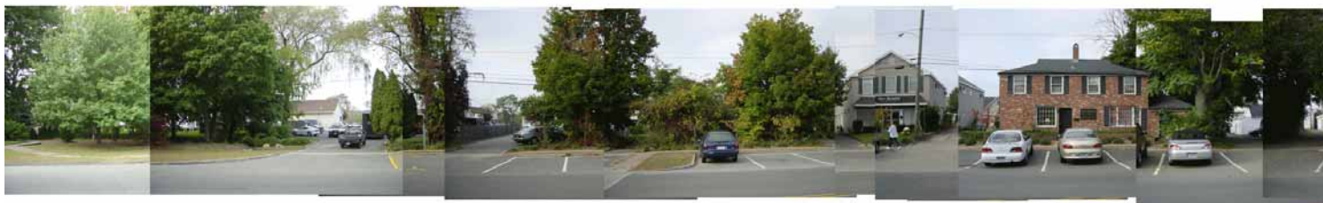
The Backs (North Elevation):
