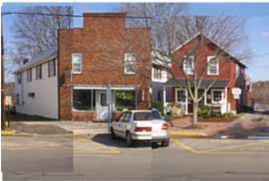
False fronts may be appropriate in the densest commercial area of Madison.
